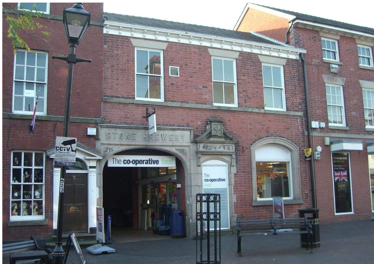
Plate 8: Former Joules' Brewery offices, High Street
