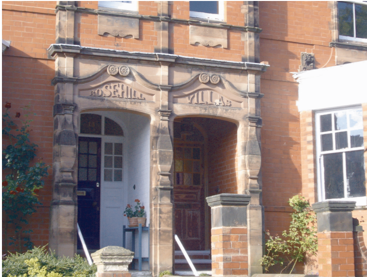
Picture 8.9 Detail of front door cases, Northesk Street
