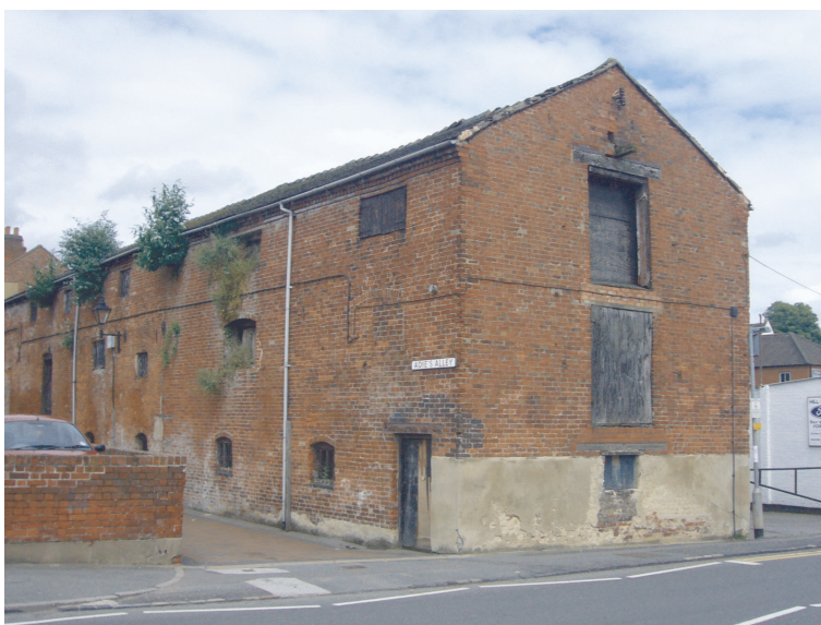
Picture 2.2 Building at Risk: Former Malthouse Adie's Alley
