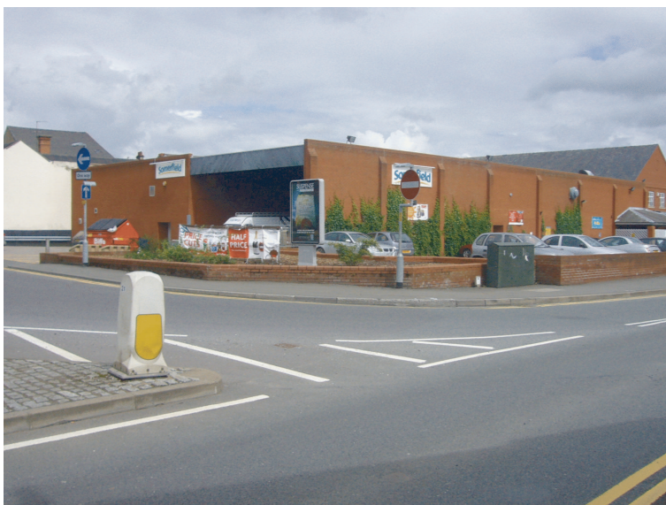
Picture 9.2 Rear of Somerfield supermarket, Crown Street
