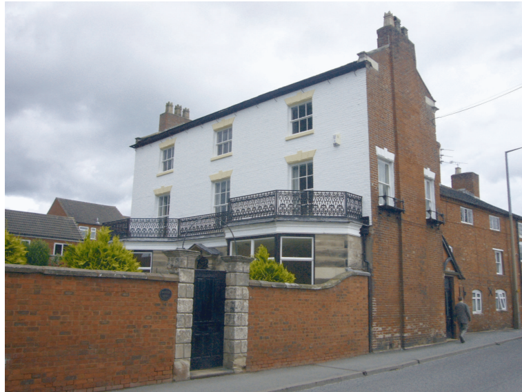
Picture 8.5 Ornate cast-iron balcony at The Mansion House, Lichfield Street
