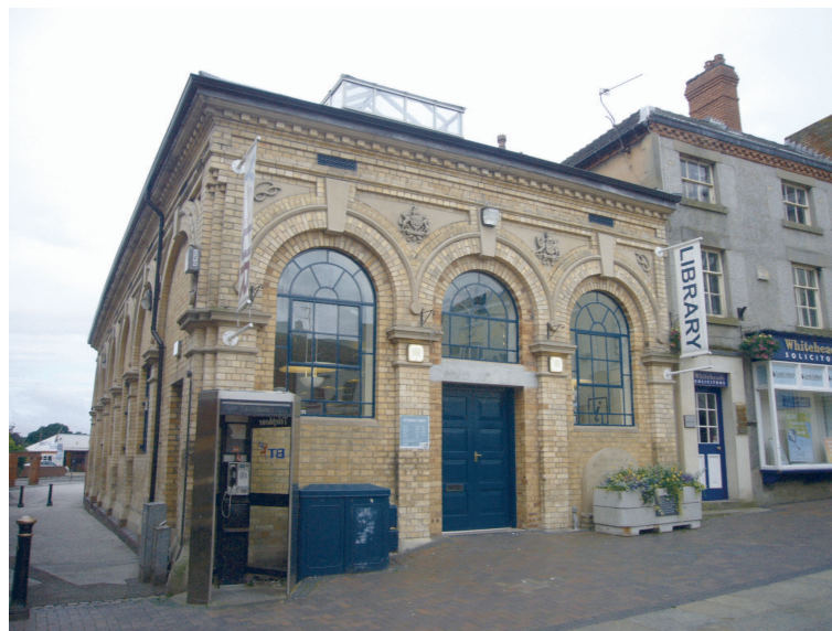
Picture 7.2 Stone Town Library - a key unlisted building
