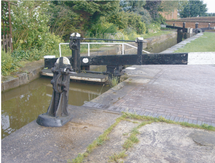
Picture 8.6 Newcastle Road lock
