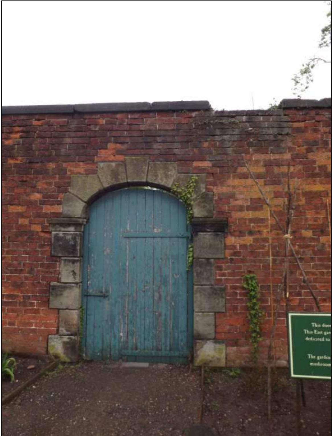
Figure 71 Eastern doorway with stepped voussoirs and plank doors with strap hinges. Copings are missing.
