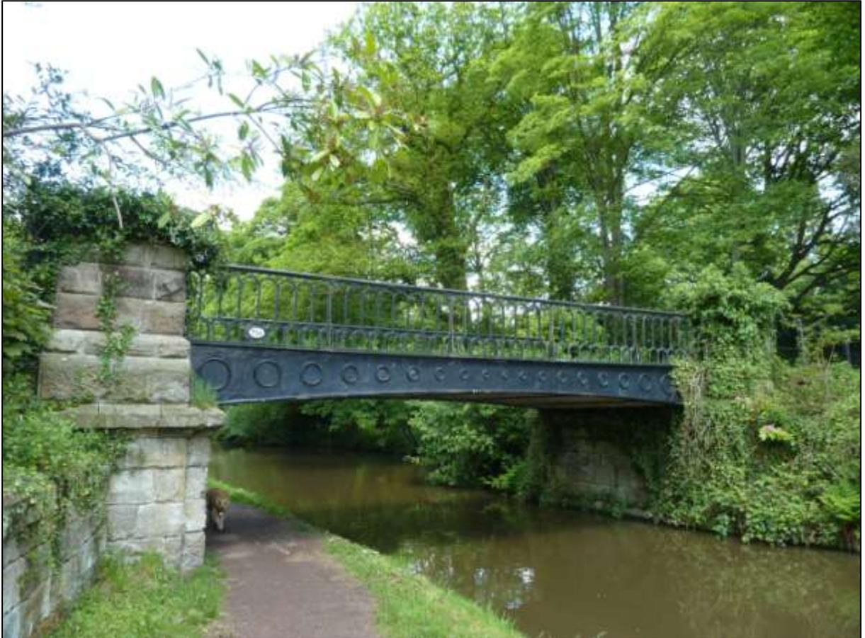
Figure 45 Iron Bridge with rusticated stone piers and circle motif on span
