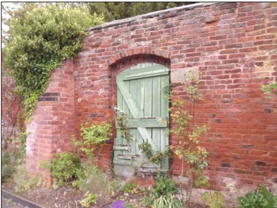
Figure 37 The continuation of Abbey House boundary wall at Abbey Gardens. The remaining plank door with original iron strap hinges is in need of repair but adds charm to the walling
