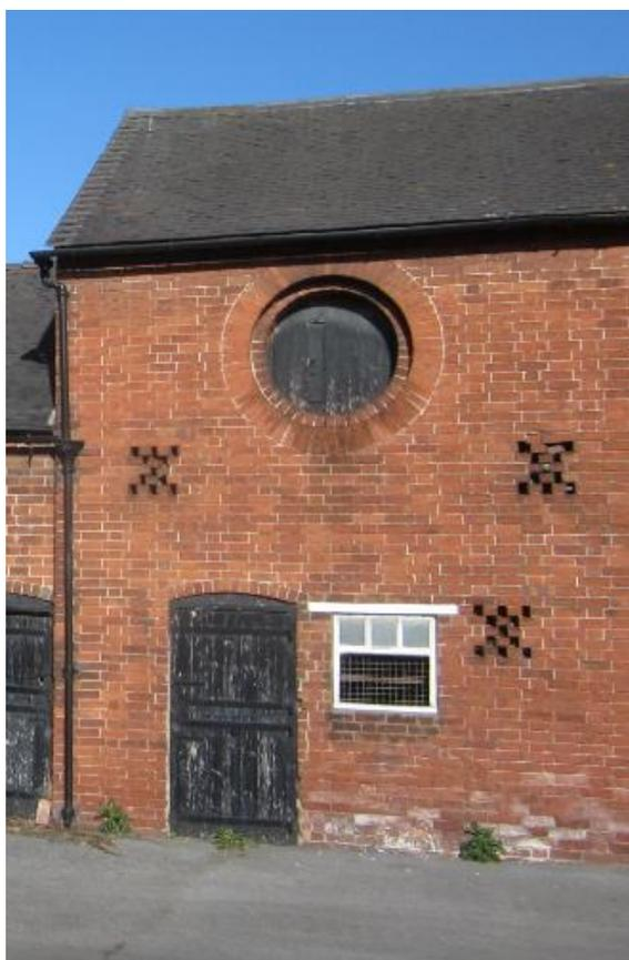
Sometimes it will be necessary to reinstate a traditional roof finish in place of a more recent alteration. This should be done in material appropriate to the locality or adjacent buildings. Natural materials should be used to repair the existing structure and avoid total reconstruction that irons out all irregularities. Much of the character of an old roof lies in its slight unevenness where it has settled between the trusses.
