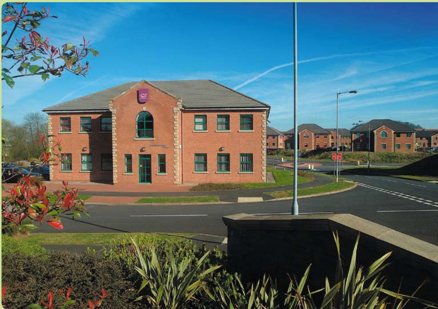
Gladmans building Staffordshire Technology Park
